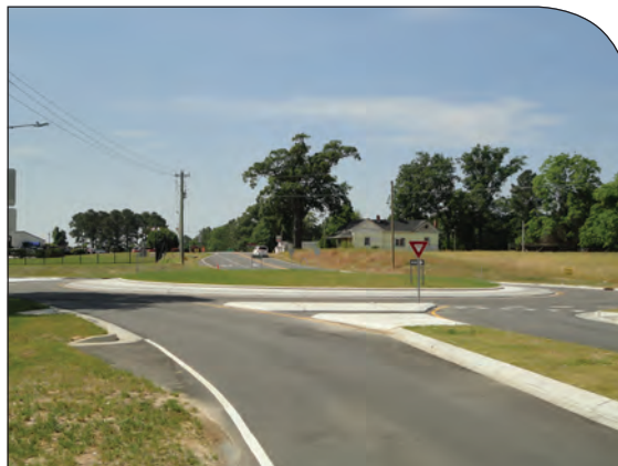
The N. Powell Avenue and N. Ashe Avenue intersection is a crash location. The road has been improved to a traffic circle since the crash occurred.
