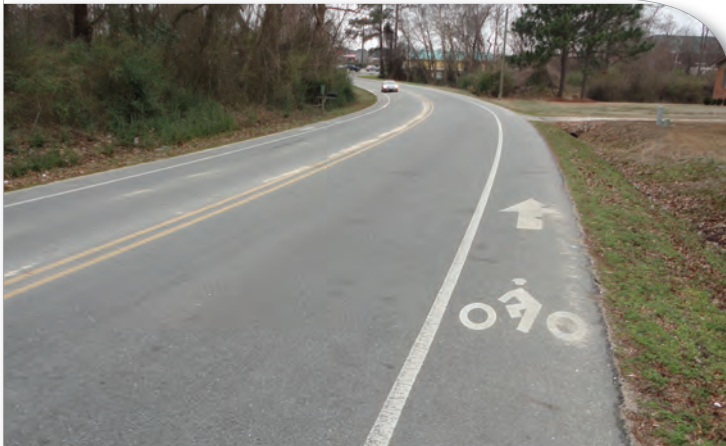
Bicycle lane on Harding Drive in Goldsboro. See Appendix A, page A-14 for bicycle lane design guidelines.
