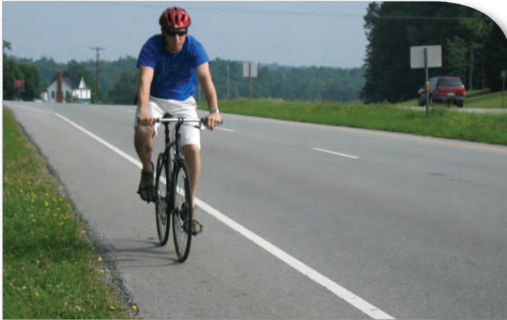
Paved shoulder in Durham, NC. See Appendix A, page A-13 for paved shoulder design guidelines.
