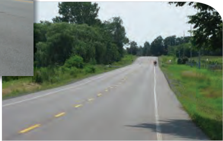
Paved shoulder, location unknown. See Appendix A, page A-13 for paved shoulder design guidelines.
