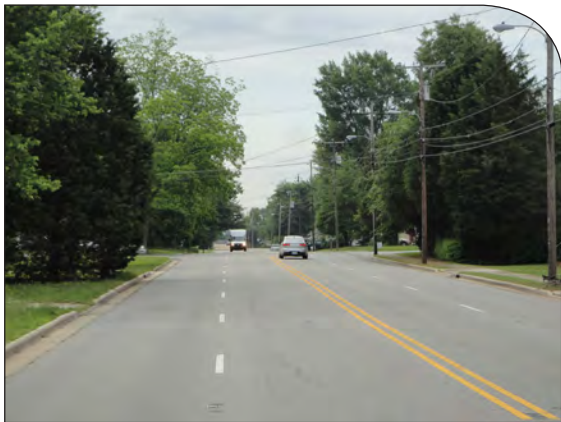
Multi-lane arterial roadways such as Pope Road are unsafe for bicyclists because of high automobile speeds and traffic volumes.
